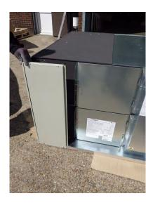
Offer up the front panel 4 to the Lossnay unit and fit using 2 x M6 X 12 set screws 12 at the base and 2 x M4 X 25 set screws 11 and 2 x nylon washers 14 to secure to the outdoor panel 3
