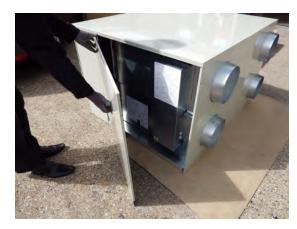
The Lossnay and weatherproof housing is now complete for final installation.
