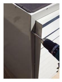
Fix the indoor 6 and outdoor 3 panels to the back panel using M4 X 25 set screws (11) and 4 nylon washers (14)
