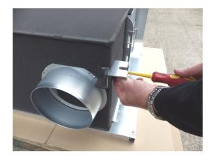
Align the back panel 6 to the Lossnay unit and fit using 3 x M6 X 12 set screws 12
