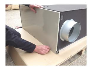
Align the OA & EA panel (5) to the Lossnay unit and fit using 3 x M6 X 12 set screws (12) and screw to the back, front and door panels using 4 x M4 X 25 set screws (10) and 4 x nylon washers (11)
